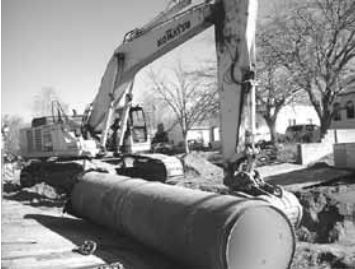
Large diameter pipeline installation.
