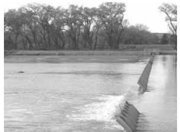
The new diversion dam on the Rio Grande.
