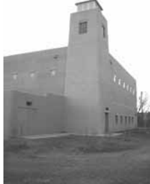
The raw water pump station.
